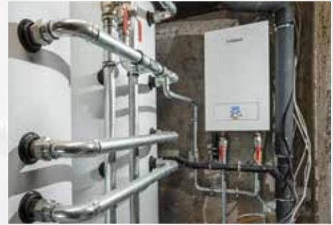
Vaillant Austria contributes know-how to the Fennerstraße refurbishment project.
