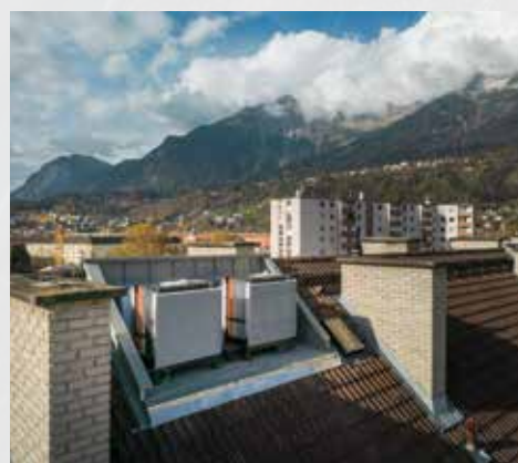
< The Vaillant aroCOLLECT heat pump outdoor unit at the time of installation work
