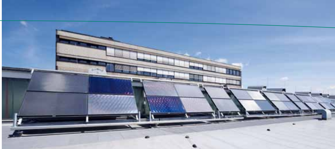
Vaillant flat-plate solar collectors ensure the hot water supply in a tube-cleaning installation at the Remscheid plant.
