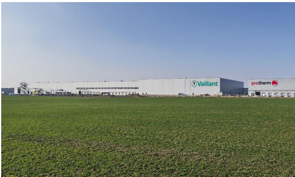
Caption: Vaillant Group's new mega factory produces exclusively heat pumps. With the new plant, the company, which also manufactures heat pumps in Germany, France and the UK, doubles its production capacity to well over half a million heat pumps per year.
