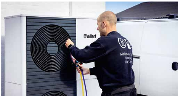
Kassebølle Friskole Reference project in Denmark (p. 34)
